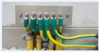
(Image of an equipotential bonding bar – these units are used to provide a convenient common earthing point within an installation)
